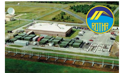
ROTHR Radar Radar Equipment Complexes
